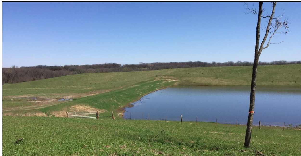
Figure 4.3. Earthen embankment of one of the Iowa Watersheds Project ponds constructed to provide flood storage.
