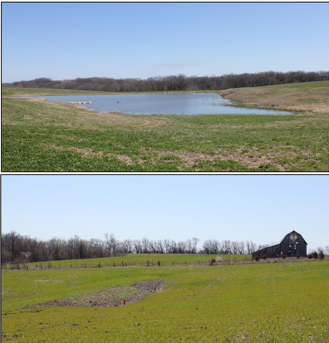
Figure 4.6. Iowa Watersheds Project Phase II project showing a water and sediment control basin.
