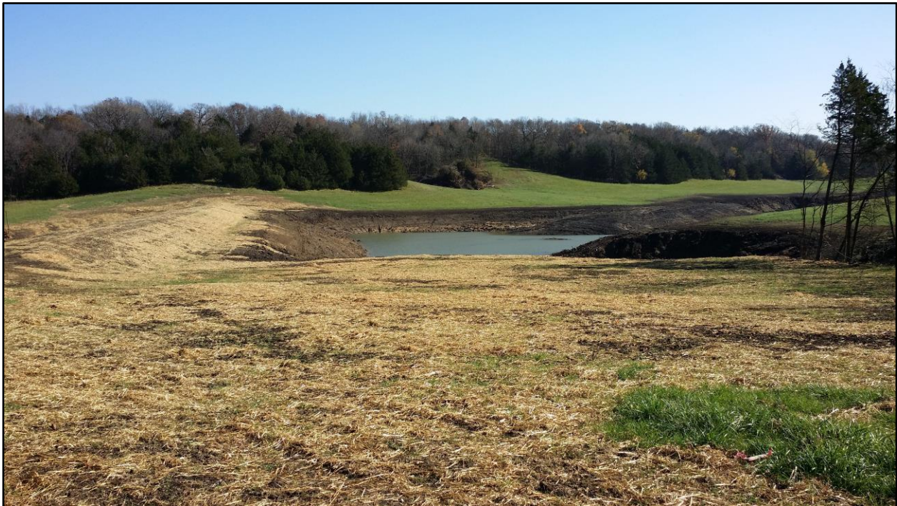
Figure 3.3. Earthen embankment of one of the Iowa Watersheds Project ponds constructed to provide flood storage.
