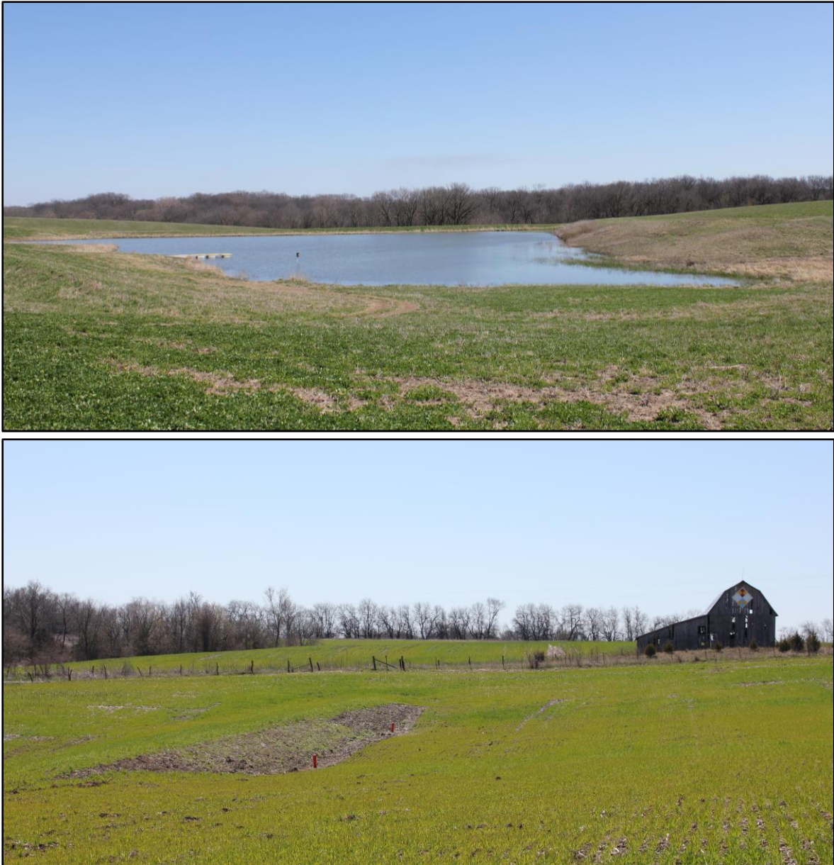
Figure 4.6. Iowa Watersheds Project Phase II projects: (top) flood mitigation pond and (bottom) terrace water and sediment control structure.
