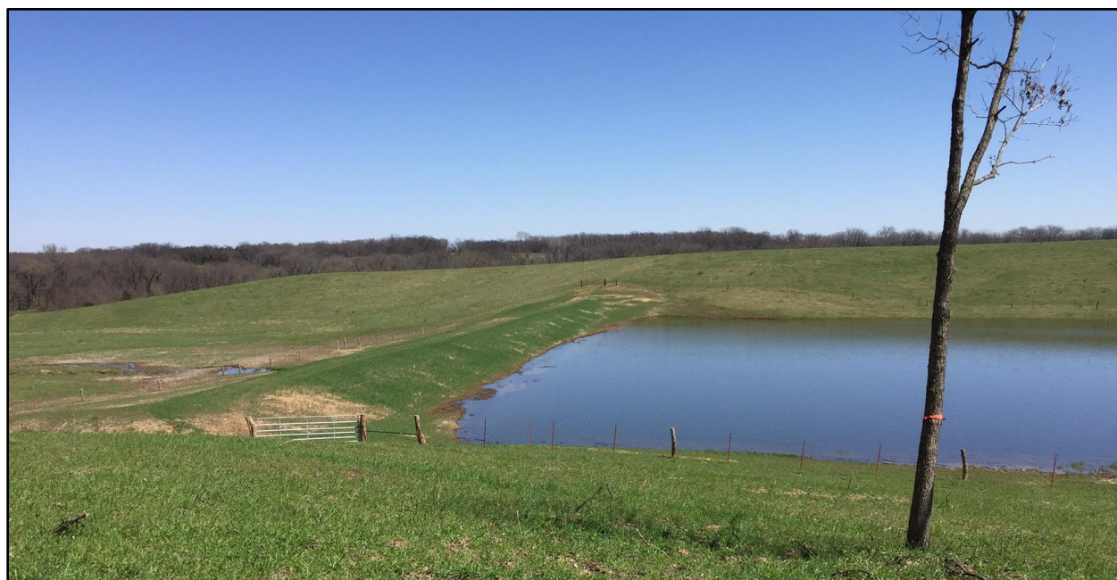
Figure 4.3. Earthen embankment of one of the Iowa Watersheds Project ponds constructed to provide flood storage.
