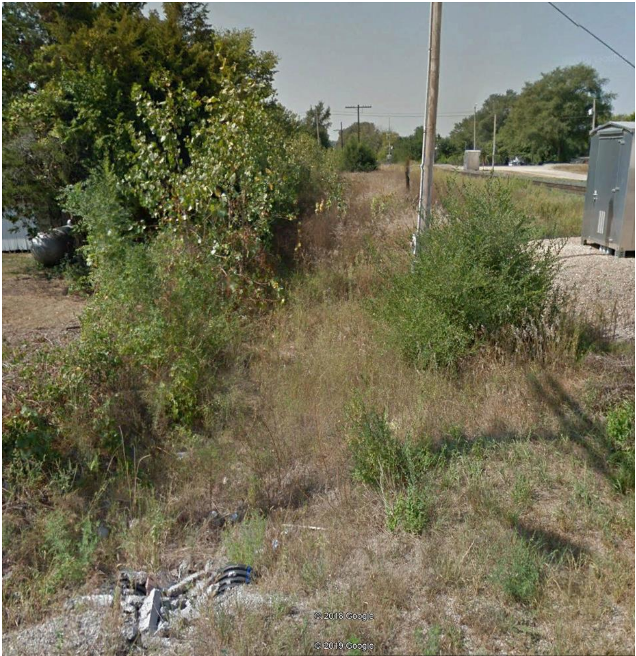
Figure 2.10. View near the intersection of 3 rd Street and the railroad, looking southwest. Twin 18-in corrugated plastic culverts convey ditch flow under 3 rd street.
