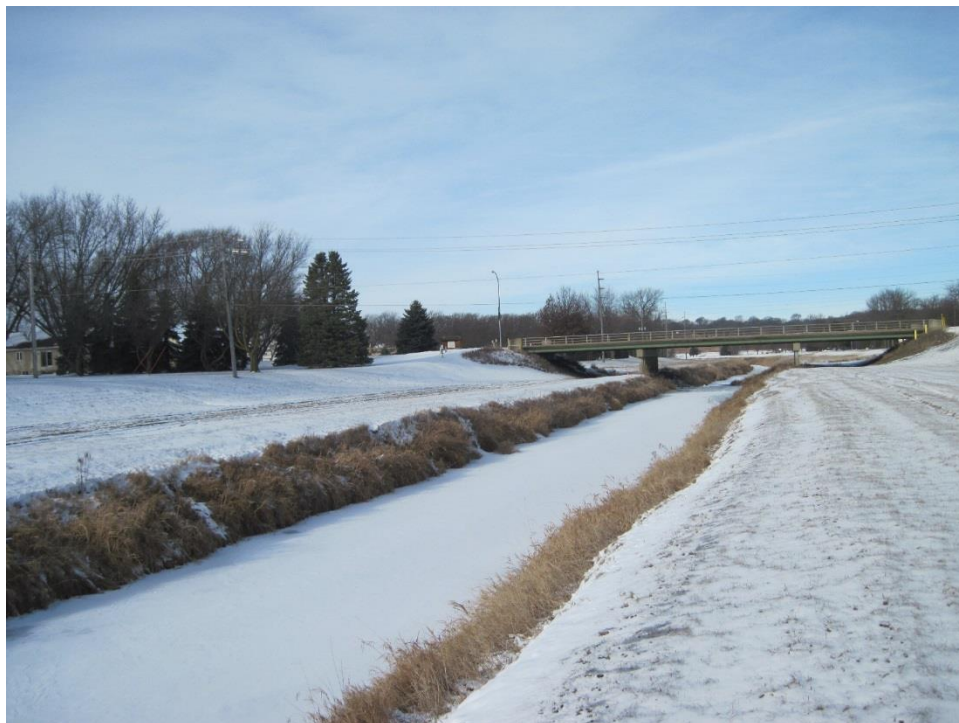
Figure 10. Typical Odebolt Creek channel conditions in downstream reach. (photo provided by JEO)
