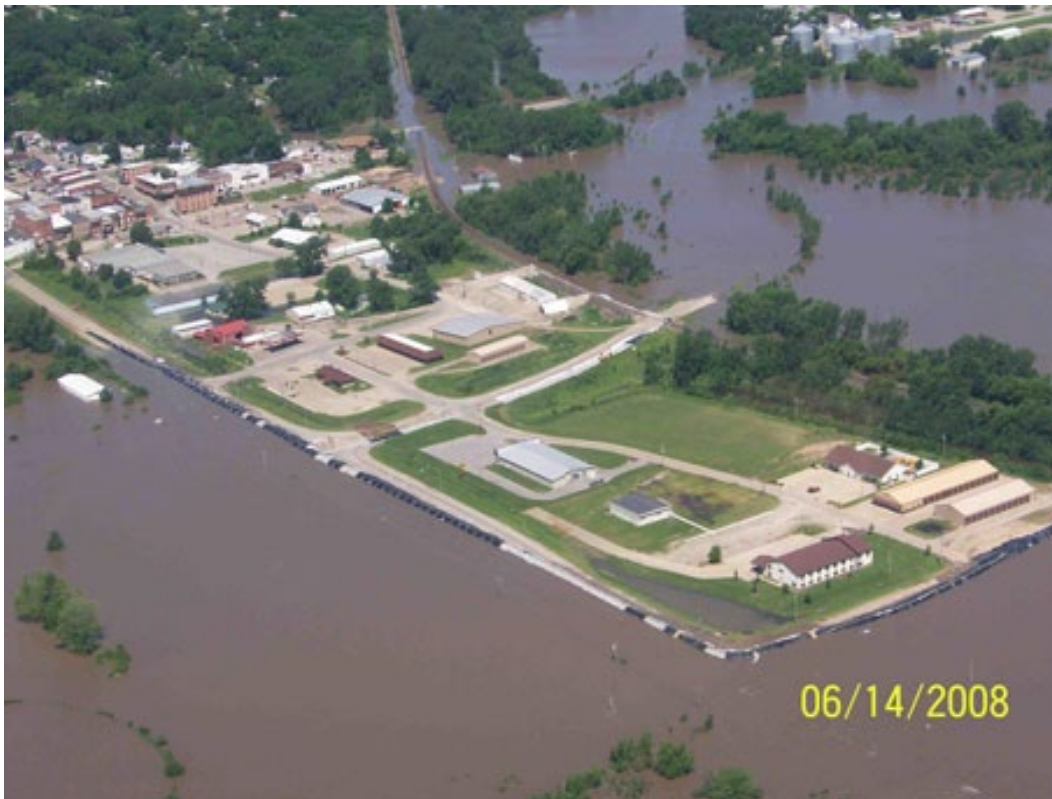
Figure 1. Columbus Junction on June 14, 2008. A temporary levee held back floodwaters until it failed, inundating several business and community buildings. Photo Credit: https://www.kenpurdy.com/FloodWeb/Flood.html
