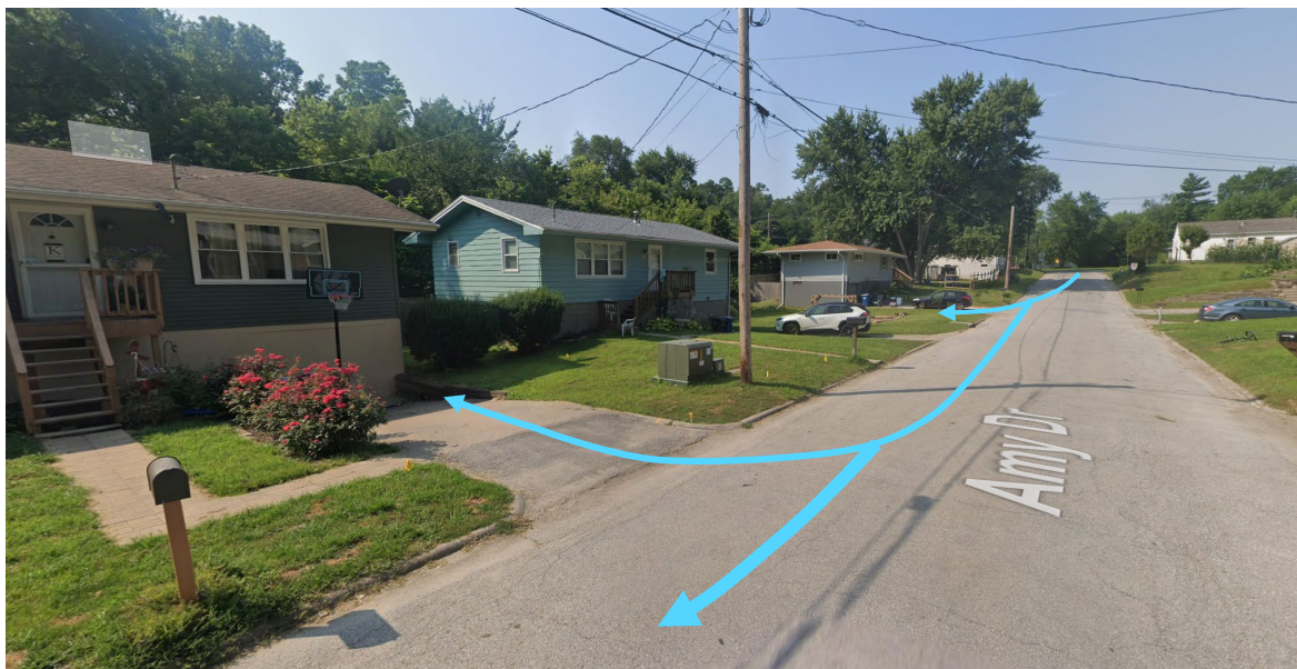
Figure 1-2. Runoff enters along the west end of Amy Drive and then enters driveways, flooding lower levels of homes.
