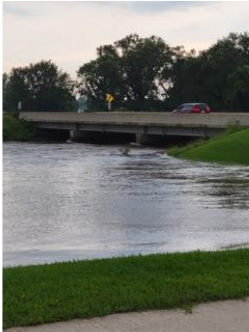
Figure 3. Crane Creek at the IA-24 bridge crossing during the August 2021 flooding event. (Photo credit: City of Lawler)
