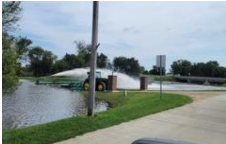
Figure 4. Flood waters in Junko Park being pumped over a small levee along Crane Creek following the August 2021 event. (Photo credit: City of Lawler)
