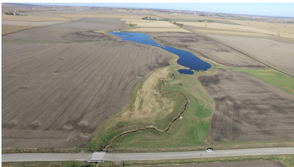
Figure 1-3: Flood mitigation wetland (MC-058 Jellison) constructed as part of the IWA in the Mud Creek HUC12, a sub-watershed of the Middle Cedar HUC8.
