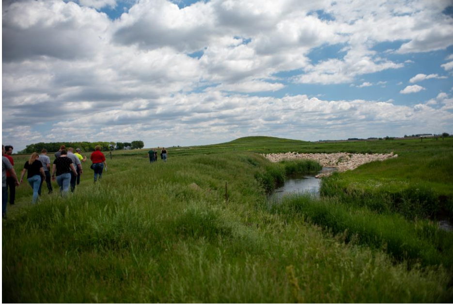
Figure 1-4: Flood mitigation oxbow and stream stabilization project (NR-001 M&M Smith Family Farm) constructed as part of the IWA in the Outlet Creek HUC12, a sub-watershed of the North Raccoon HUC8.
