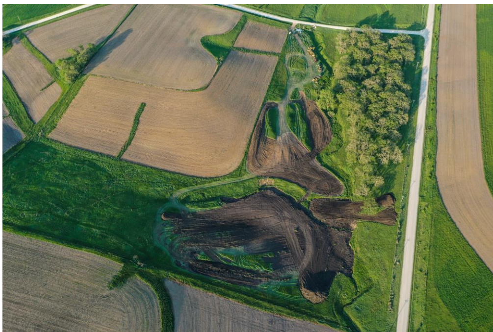
Figure 1-3: Flood mitigation pond (UI-039 Branhagen) constructed as part of the IWA in the Community of Nordness HUC12, a sub-watershed of the Upper Iowa HUC8.
