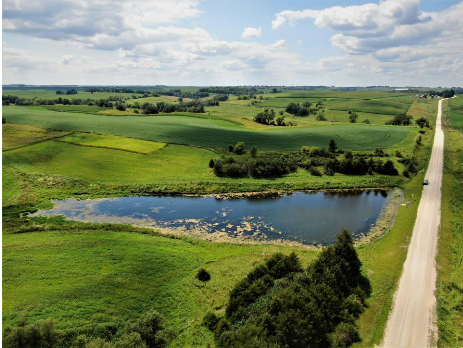
Figure 1-4: Flood mitigation on-road structure (UI-022 Weselmann) constructed as part of the IWA in the Trout Creek HUC12, a sub-watershed of the Upper Iowa HUC8.
