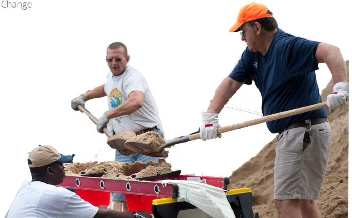
Figure 3.1 Flood 2013 Source: University of Iowa
